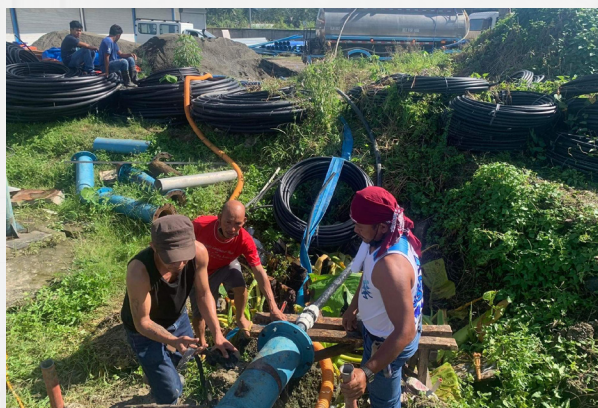
BCWD personnel ensuring that the tapping point for the water tankers is not leaking.
